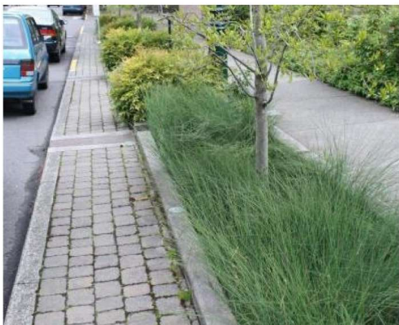
Figure 41: Green Street with swale
